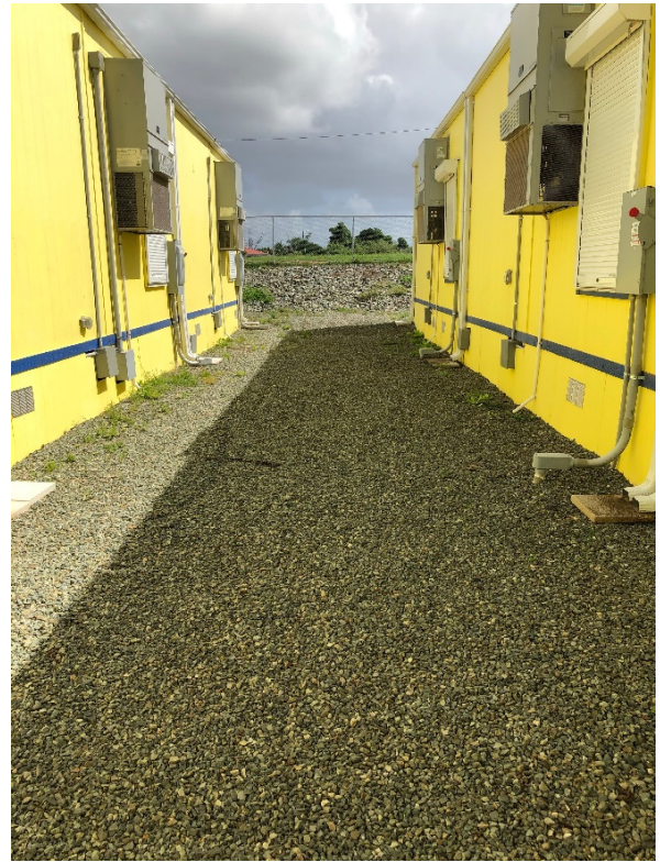
Several Downspouts leading to French Drain system
